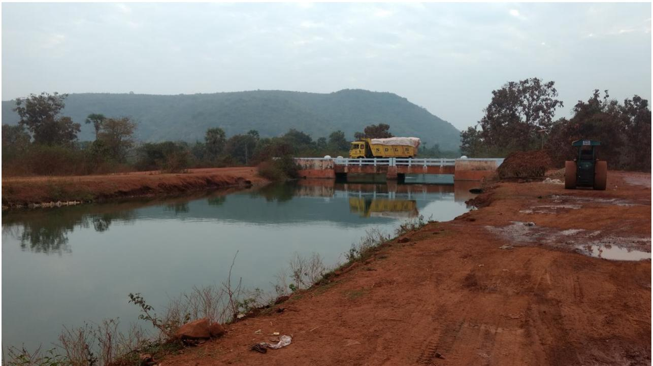
Figure 13: trucks carrying heavy loads crossing the bridge which is only constructed for villagers to cross and does not have the capacity to take 300 heavy loaded trucks every day
